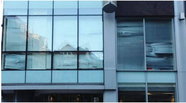
Figure 3.3 Internal venetian blinds poorly retrofitted into a new building in London.
